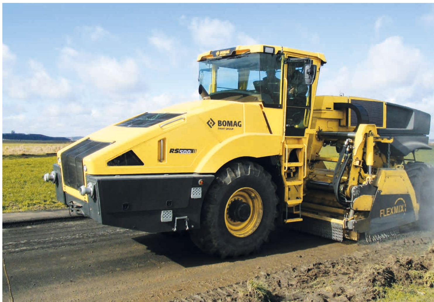
Milling 8 cm of asphalt road.
