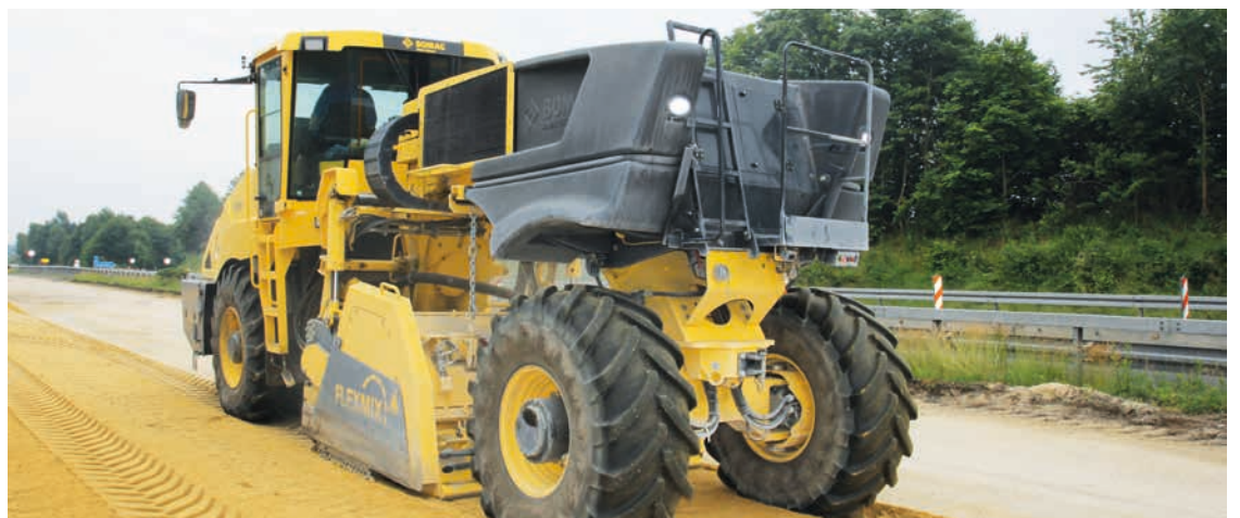
Milling a hydraulically bound base course.
