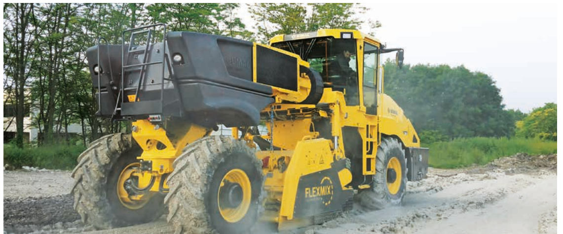
Homogenisation of cohesive soils to a 50 cm depth.
